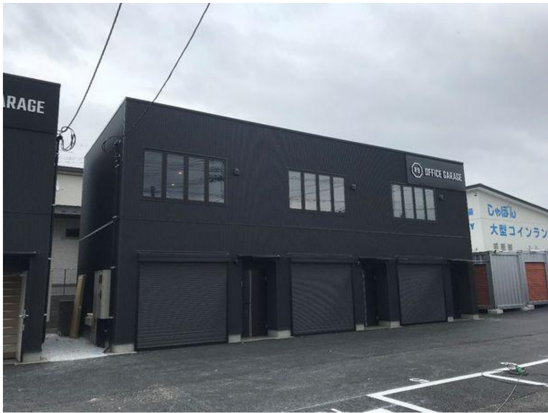
R9 OFFICE GARAGE藤岡(2)
