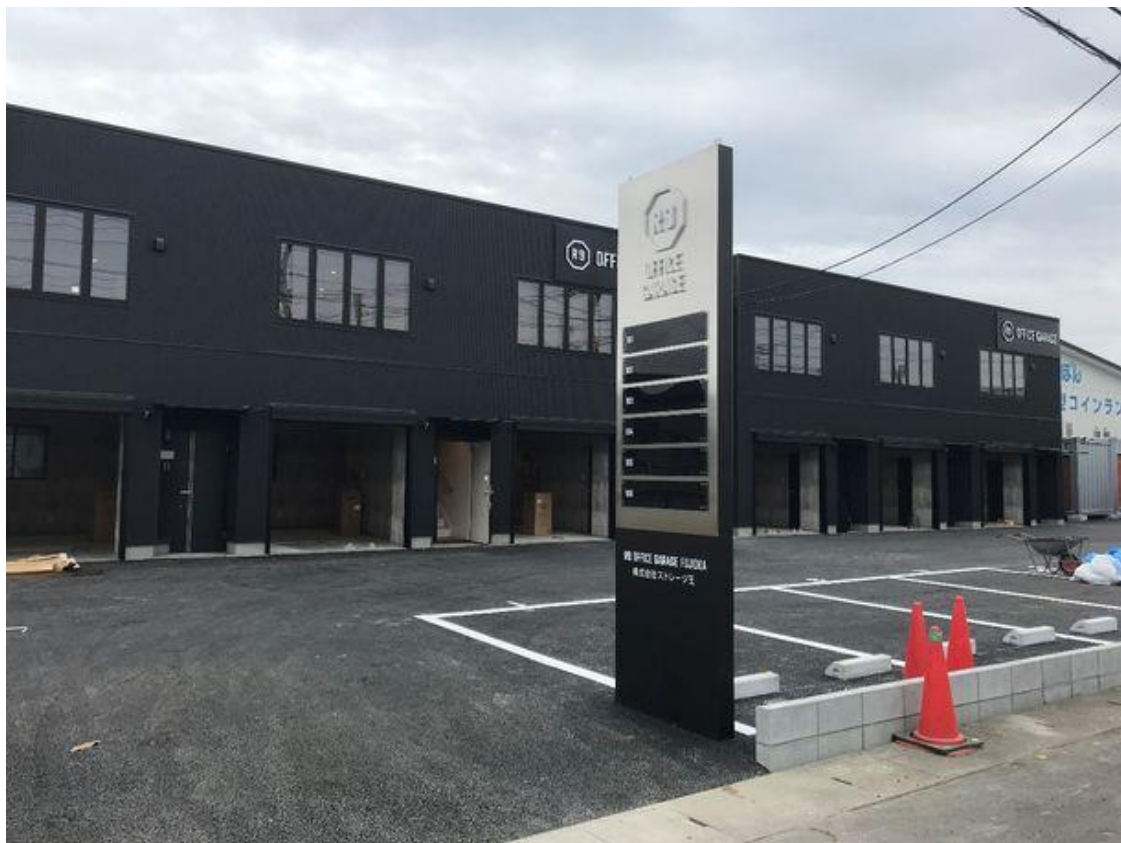
R9 OFFICE GARAGE藤岡(1)
